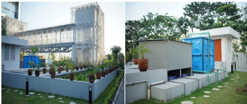
Fig. 4. Waste Water Treatment
